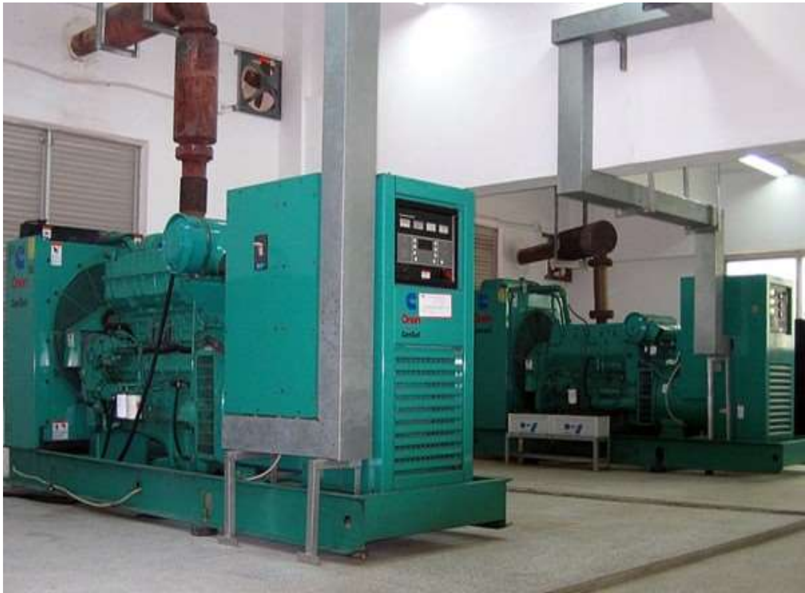
Electricity generators – 1MW to support entire plant
